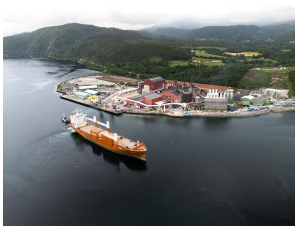
Figure 32 - Wacker Chemicals Norway's silicon metal plant at Holla. (Photo: Wacker)
