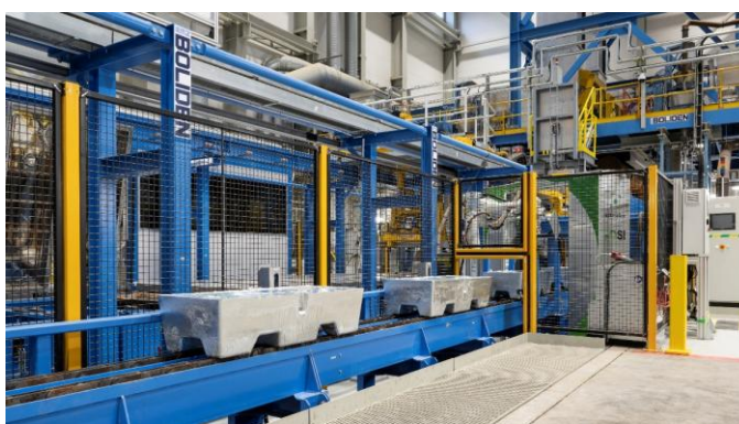
Figure 28 - Transport of cast products at a fully automated zinc foundry at Boliden Odda. (Photo: Thor Brødreskrift)
